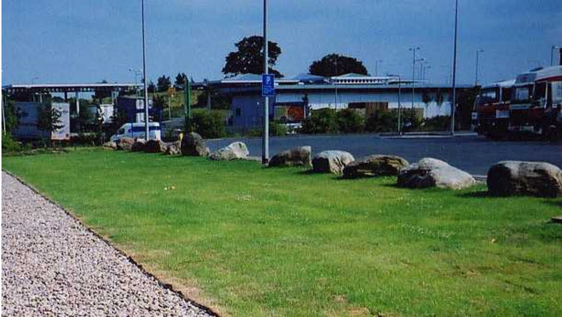
Figure E1-19 Filter Strip, Hopwood Services, UK
