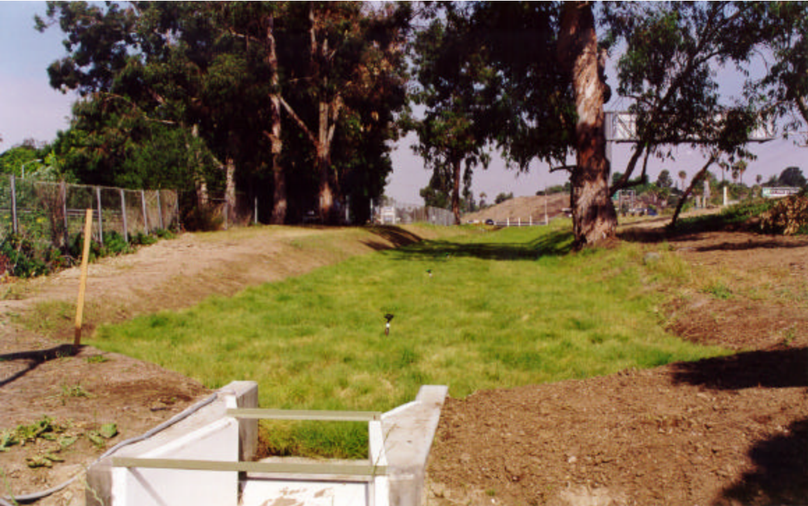
Figure E1-11 A Vegetated Swale along I-15, San Diego County
