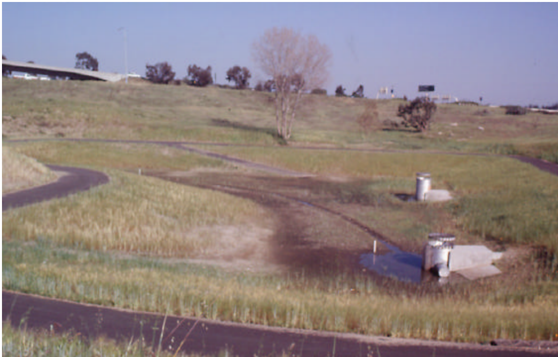
Figure E1 -1 Dry Detention Basin, I-15/I-78 Intersection, San Diego County
