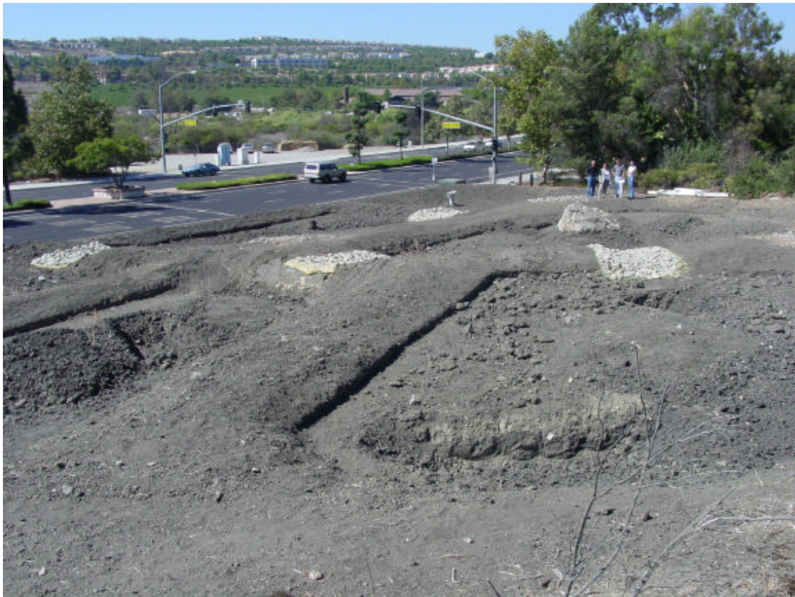
Figure E1 -36 North Wetland under Construction
