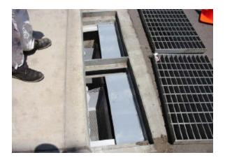
Figure 3-15 BioClean<sup>™</sup> Insert
