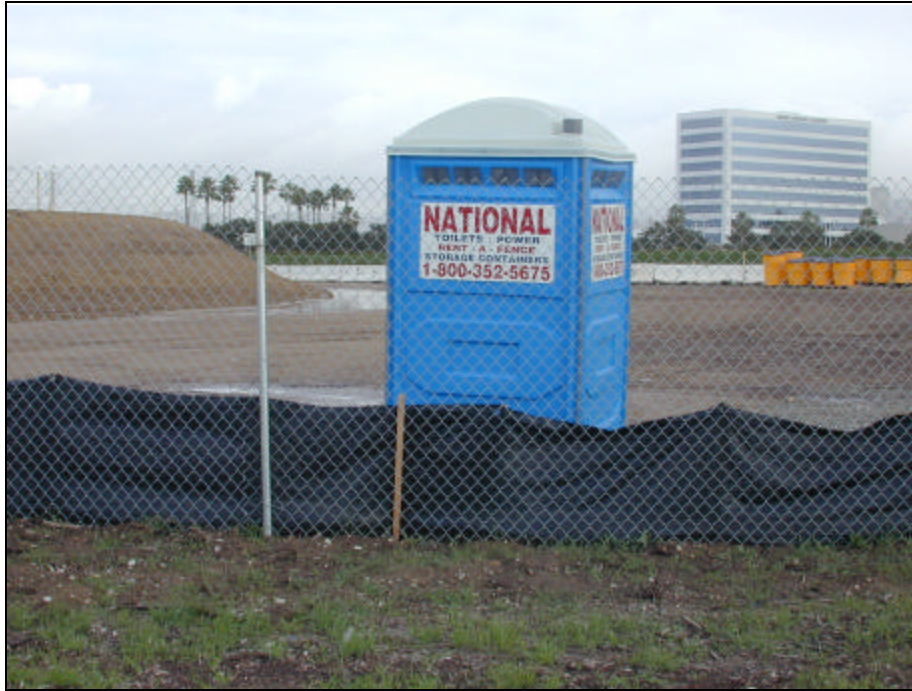
Figure 2-2 Portable Toilet Placement at a Construction Site
