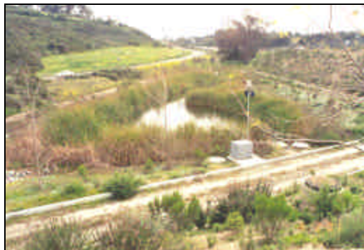
Figure E6-14. Typical Wet Pond
