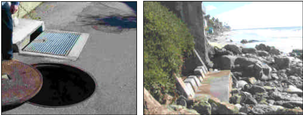
Figure E6-13. Cleo Street at Gaviota Drive CDS™ Diversion and Beach Outlet
