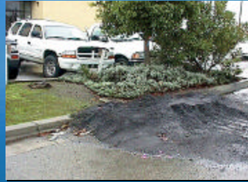
Stockpile should be relocated, covered and protected from run-on
