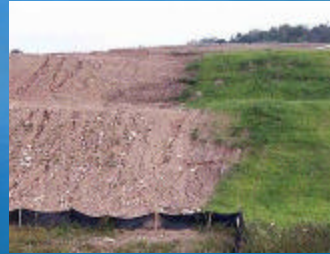
Unstabilized slope vs. Stabilized slope
