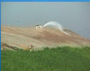
Soil binder applied via water truck
