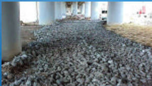
Large diameter rock used as a stabilized entrance / exit.
