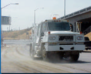
Street sweeping and vacuuming
