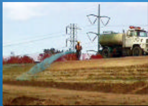
Application of Soil Binder
