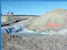
Below Grade concrete washout
