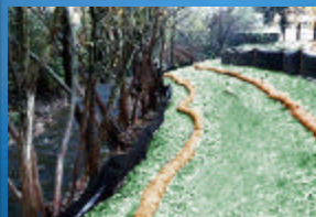
Correct installation of fiber rolls
