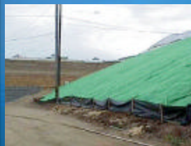
Erosion Control Blankets
