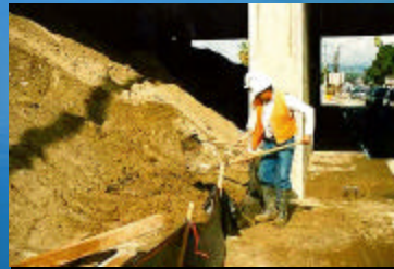
Silt fence maintenance
