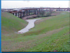
Hydroseeded slopes show vegetation growth
